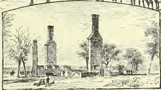
RUINS OF THE WHITE HOUSE, WHICH WAS BURNED JUNE 28, DURING THE "CHANGE OF BASE."
